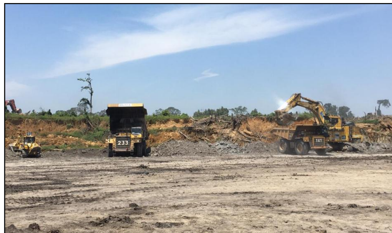
Gambar 6. Proses Loading Soil Rawa dan Layerig Material Overburden
