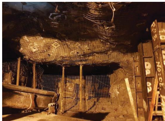
Figure 8. Rehab activity of Panel 03
