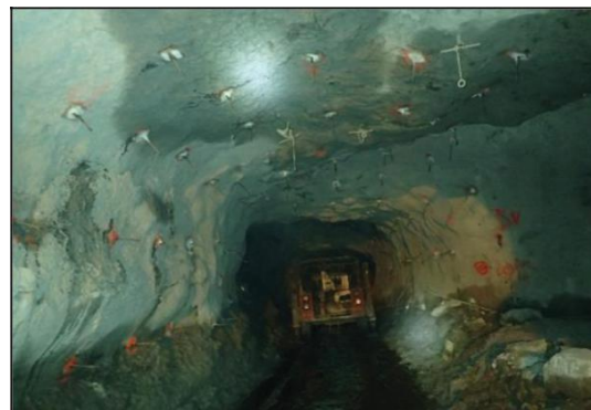
Figure 9. Rehab activity of Panel 1H
