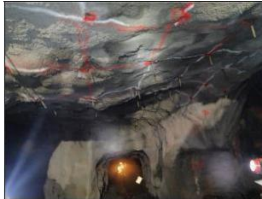
Figure 7. Rehab activity of Panel 04
